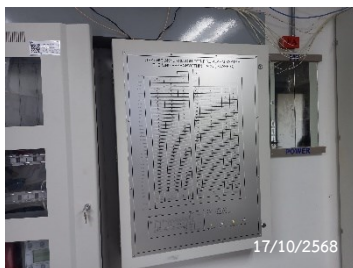
Graphic Annunciator Fire Alarm System
