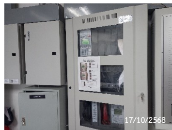
Fire Alarm Control Panel
